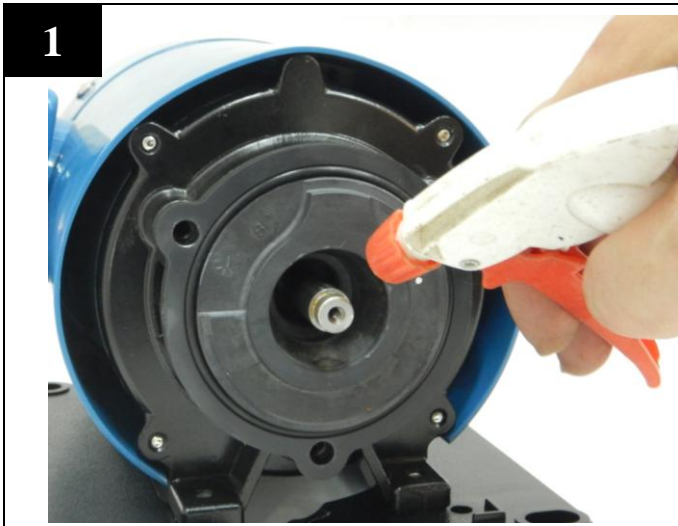
Spray water on the shaft as lubrication.
